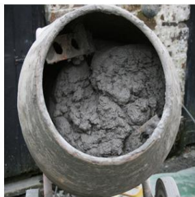
Fig.6.1: Mixing of all ingredients for preparation of concrete
