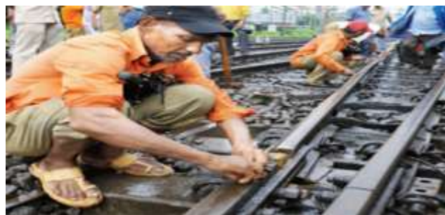
Figure 2: Traditional Railway Track Crack Detection.
