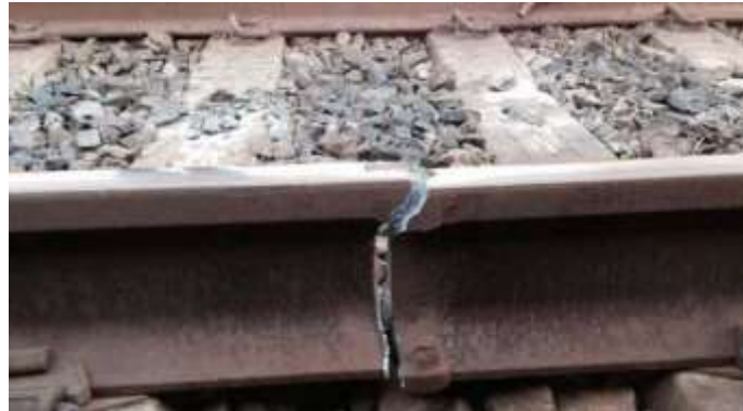
Figure 1. Crack in Railway Track.
